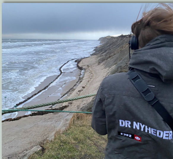
FEBRUARY 2020 – ONE ROW OF FASCINES NOW HIDDEN BY NEWLY TRAPPED SAND.
