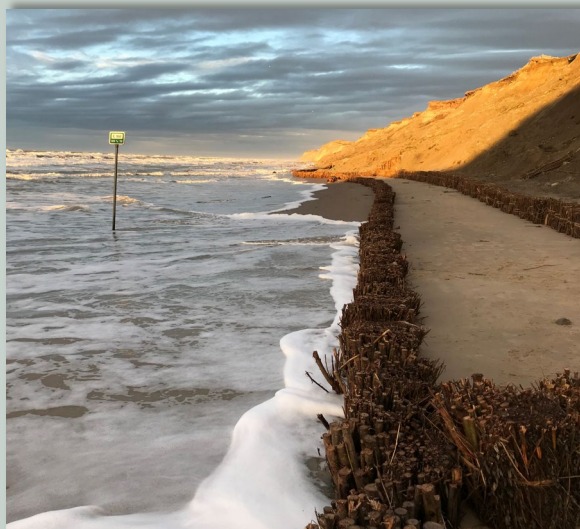
DECEMBER 2018 – WINTERSTORM, FASCINES ABOVE TERRAIN
