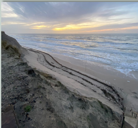
JANUARY 2020 – FASCINES ARTLY COVERED - FOLLOWING THE NATURAL LANDSCAPE COASTLINE
