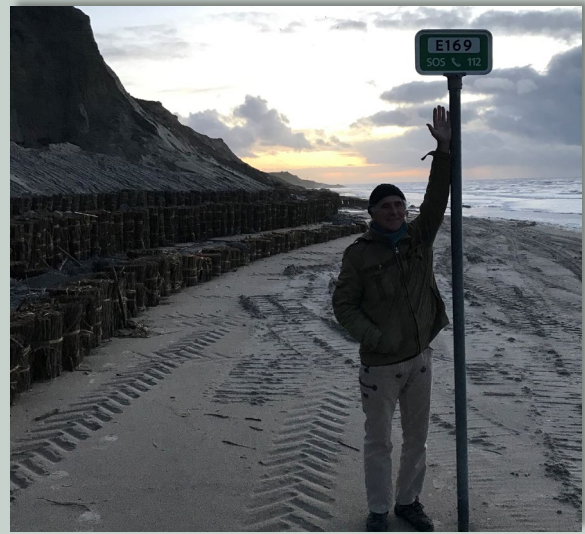
DECEMBER 2019 – FASCINES PARTLY COVERED
