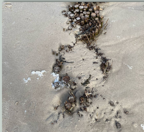
FEBRUARY 2020 – FASCINES ALMOST HIDDEN
