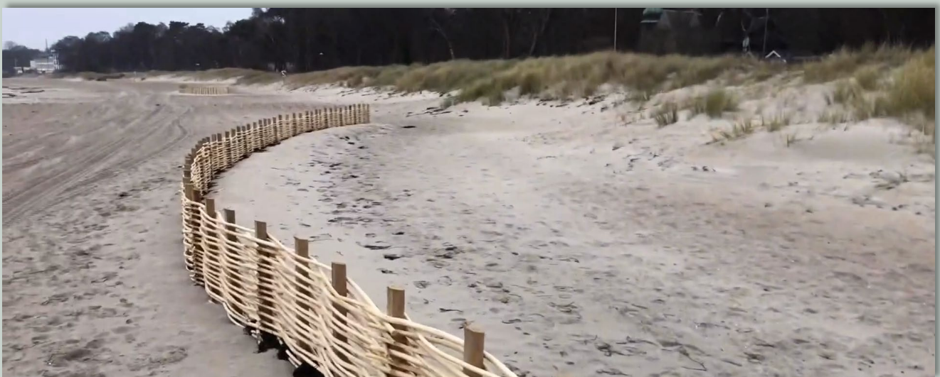
Hurdle applied as sandtrapper at YSTAD Municipality (Sweden) – part of the LIFECASTADAPT Program.
