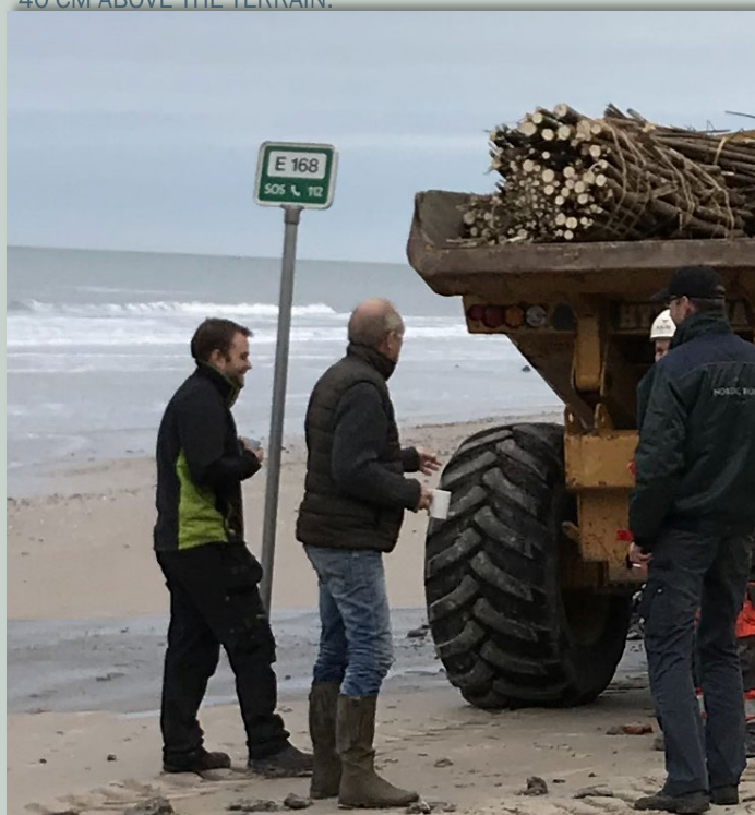
THE PLANT HAS GAINED SAND FROM THE SEA AND SURROUNDINGS FOR 9 MONTHS. THE BEACH HAS BEEN RAISED DURING THIS PERIOD, AND FACHINES NOW ONLY 5-15 CM ABOVE TERRAIN.
