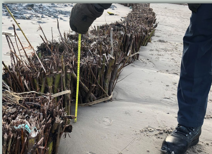
THE BEACH HAS BEEN RAISED AFTER MILD STORMS AND FASCINES NOW 30 CM ABOVE TERRAIN.
