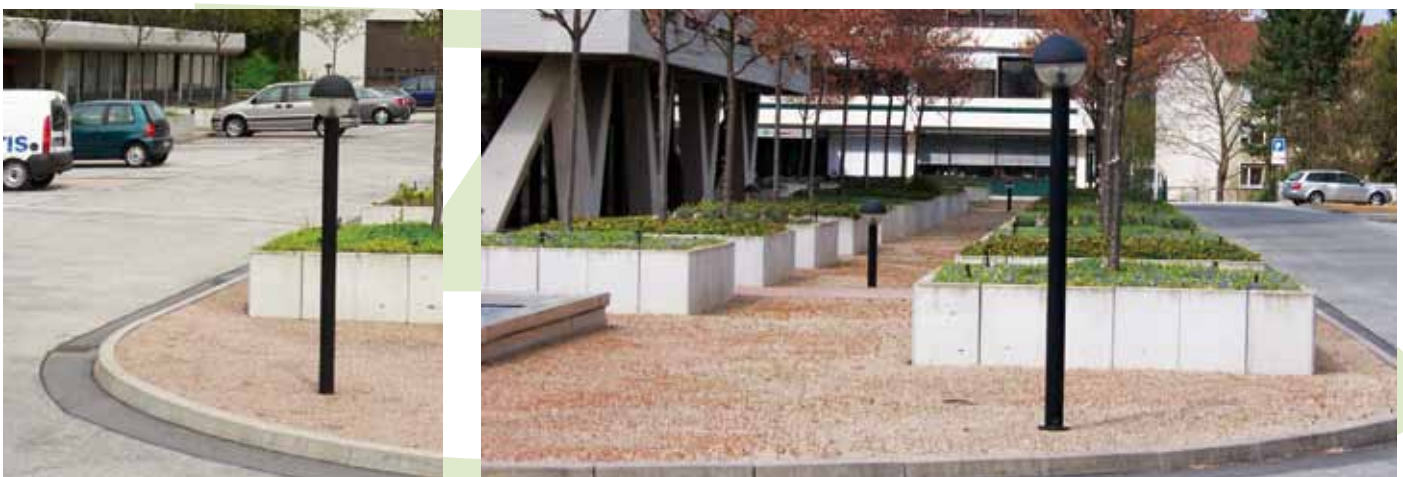
A continuous drainage layer based on Floradrain® FD 60 has been realized both below the planters and below the driveway.
